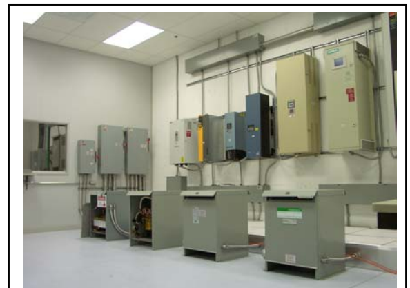
Figure 16-1: H&E Lab showing Non-linear Load Bank
