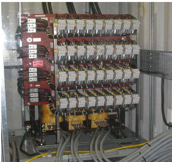
Fig. 18. One of two 750kW Lineator™ units installed on each group of 750kW combined thruster and pump load
