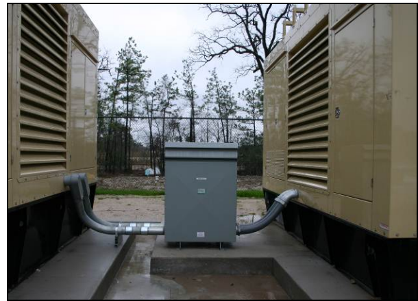
Figure 9: Photo of GenLink DPNL installation
